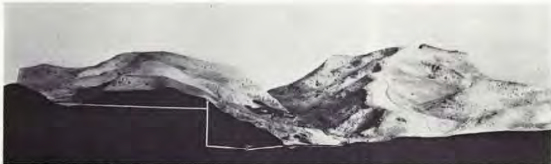
A cut-away model of the proposed Dinorwic scheme showing the water tunnel leading from the upper reservoir, left , to the power station and then to the lower reservoir.
