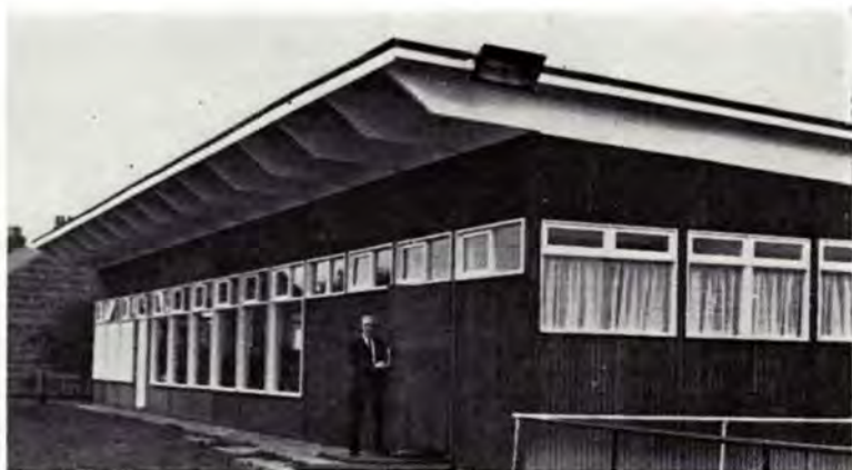
The familiar office block now on its new site. In the doorway is Mr. Ken Wynne.
